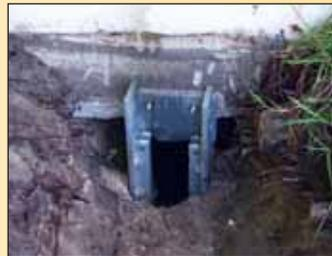
3. The pier is hydraulically advanced to the required depth while the home is monitored for movement.
