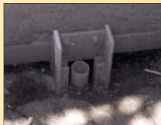
The excavation for the pier is typically not much larger than the bracket, and therefore is performed by hand.
