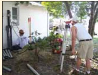
4. After the foundation is stabilized and leveled, the pier is locked in place on the bracket, trimmed, and covered with the excavated soils.
